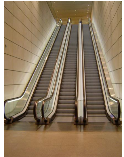
RFID tags on escalator steps makes it easier to forecast potential failures.
